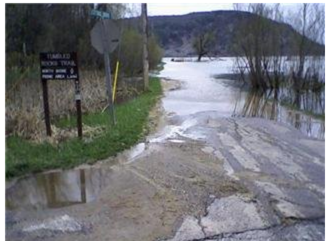
Devil's Lake spreads past its shoreline covering part of the road leading to the cabins and Tumbled Rocks Trail. April 26, 2008. Photo courtesy of Todd Cornilsen.
